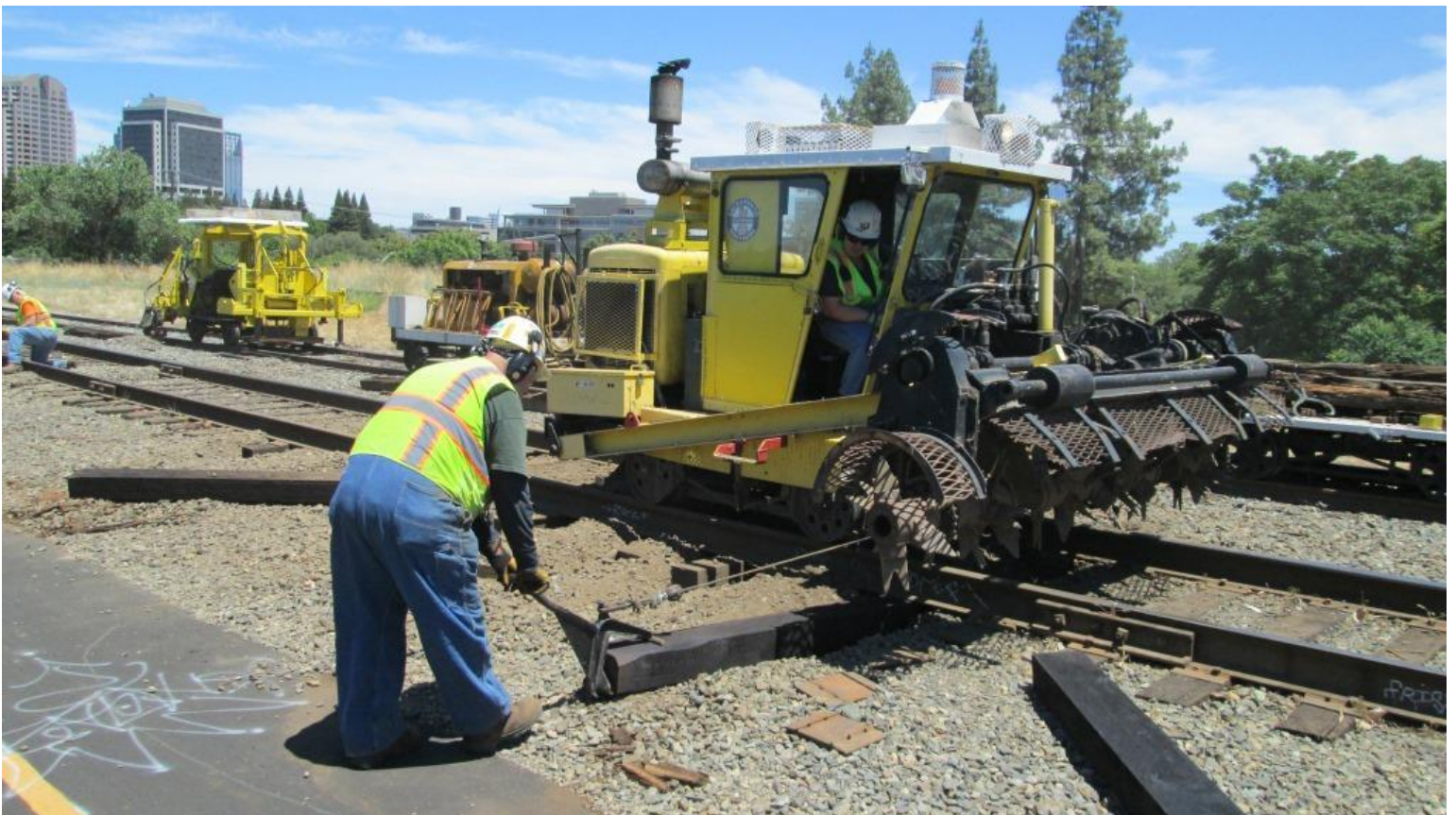
Mike guides a tie as Heather as Heather in the scarifier pulls it into place
