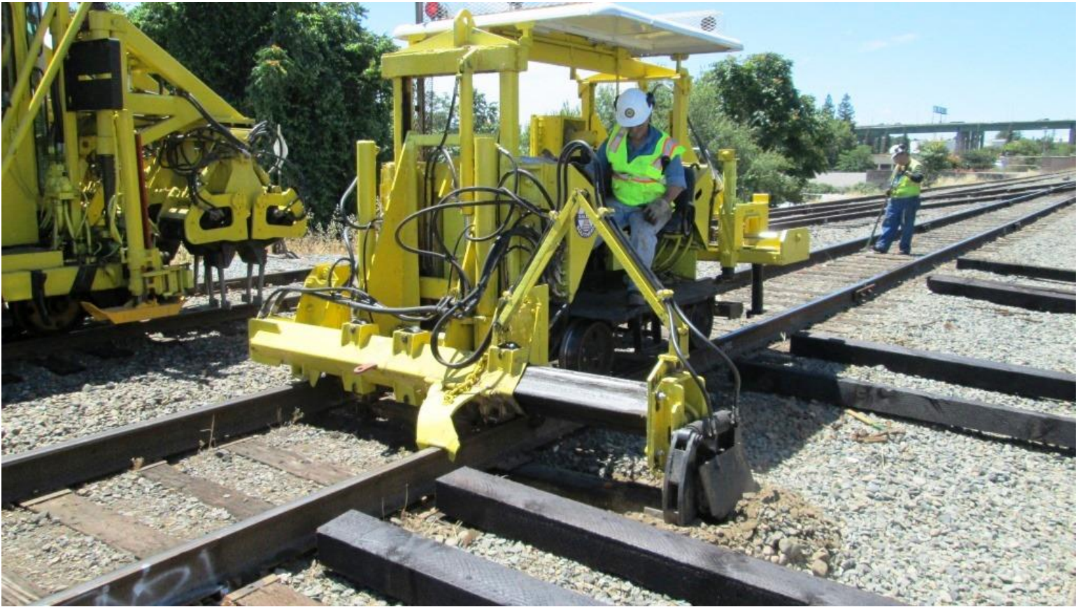
Joe on the 125 carefully shimmies-out a tie before it crumbles to dust
