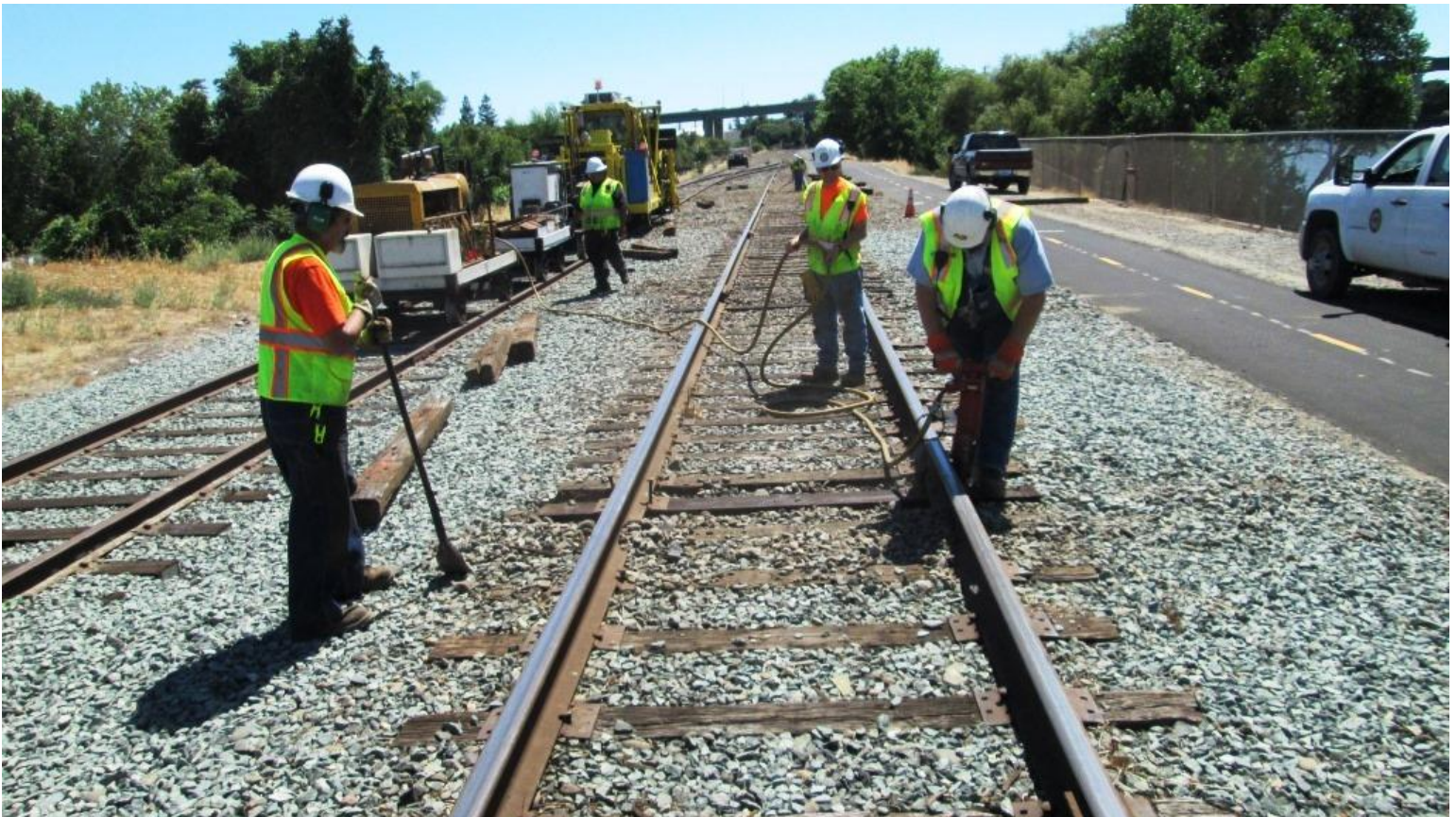
Ed stands ready with the nipper as Mike W. guide the air hose as Chris drives spikes
