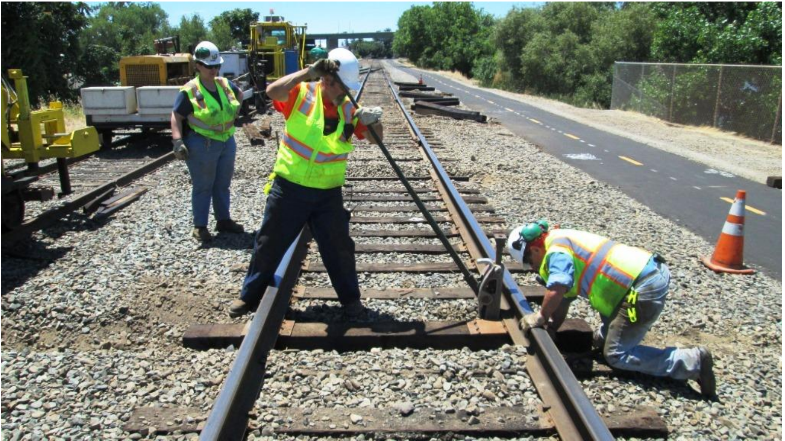
During lunch, Heather, Ed, and Joe continue working by jacking-up the rail to insert tie-plates
