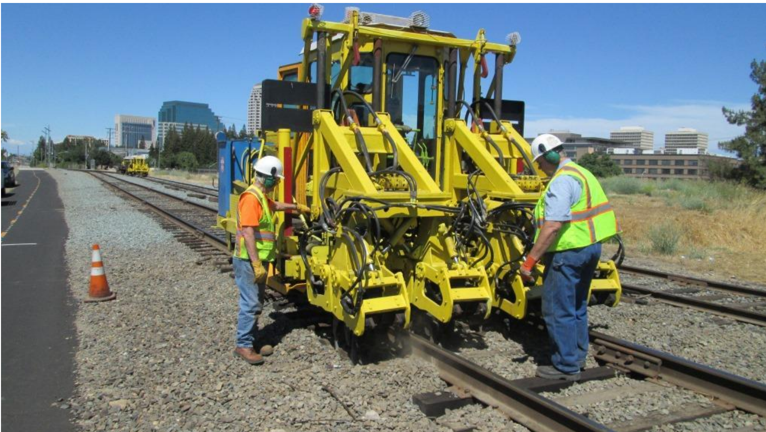
Tamping was the final act of the day. Chris directs Mike F. in the tamper as Mike W. actuates the squeeze mechanism
