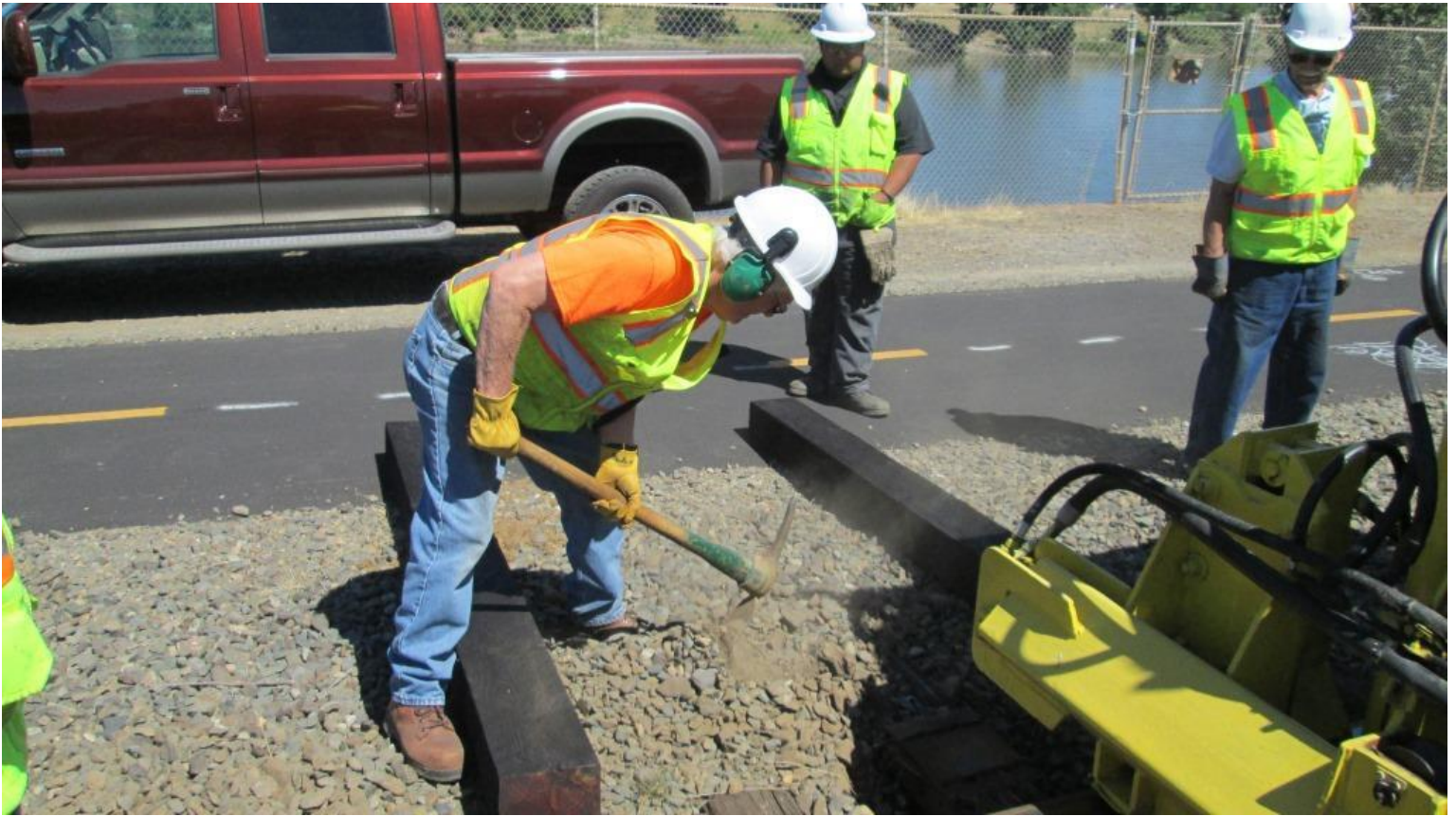
...As Mike W. clears rock away from the tie's direction of travel
