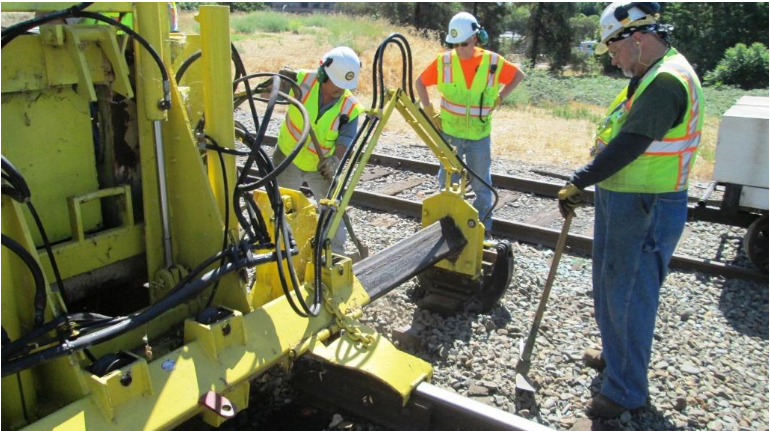
Joe and Mike F. dig around the end of the tie so that that the ram will be able to push up against the tie squarely
