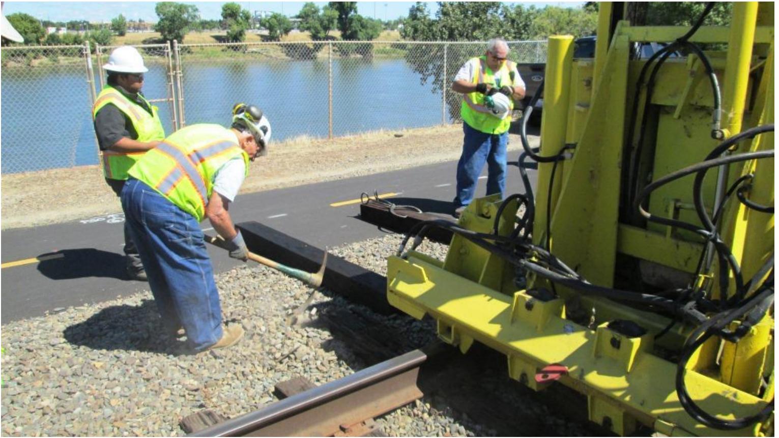
Clem digs out the other side in order to give space for the old tie to be removed without it turning to splinters
