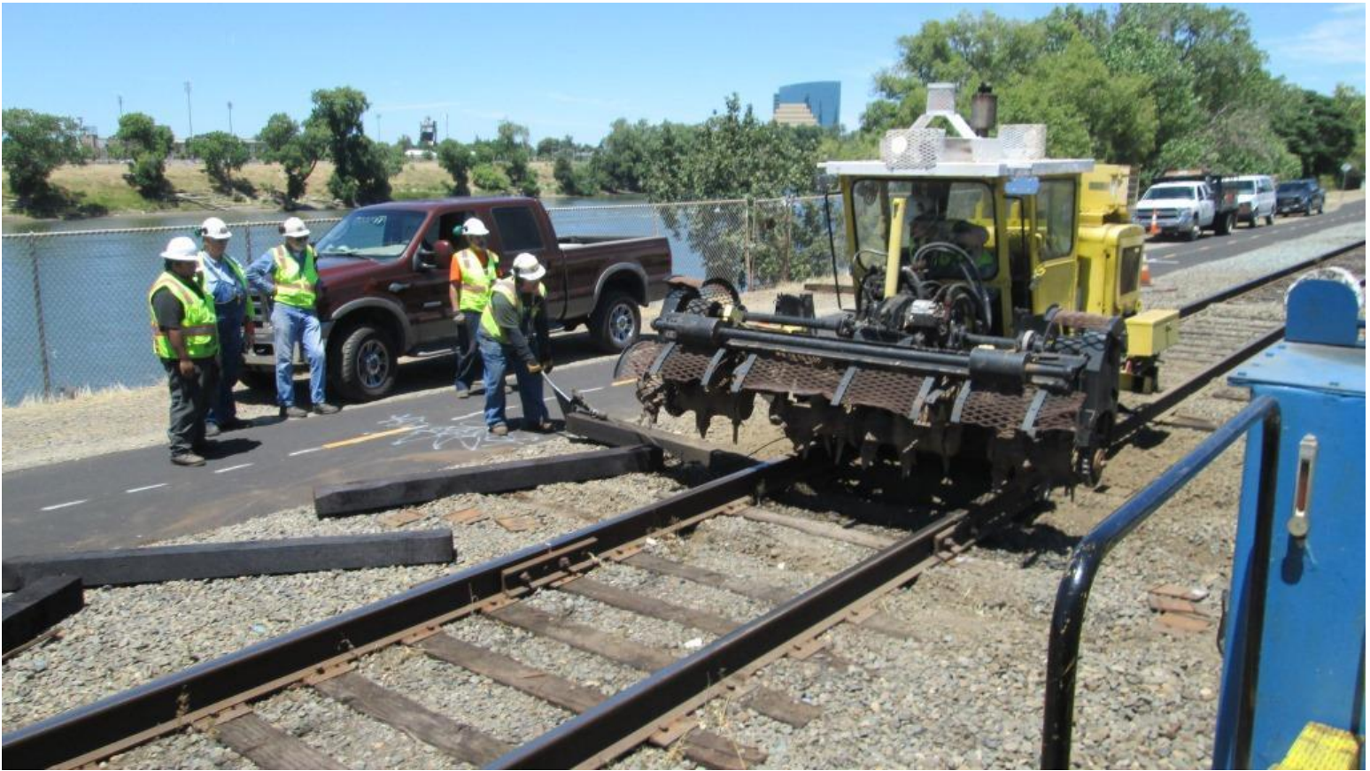
The last few ties are inserted
