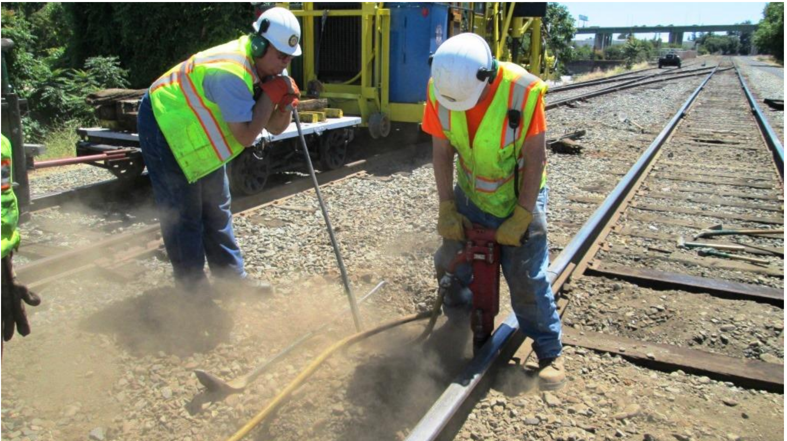
Chris nips-up the tie as Mike W. uses the pneumatic spike-driver to drive a spike
